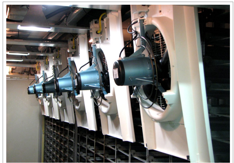
Heating element and humidity system mounted to plastic fan board
