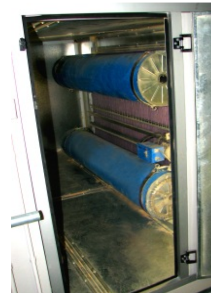
Hatcher duct mounted automatic roll filter
