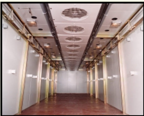
Bio-secure Design: Clear floor area allows the entire machine to be cleaned easily and efficiently during the setting cycle. Extra humidity spray points are mounted in the impeller fan boards above the central corridor.
